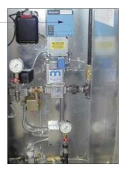
Reactivation temperature sensors are 500°F rated Platinum thermistors. The units use combination circuit breaker/overload/ starters for fan motors. This eliminates the need for spare power fuses, and saves the customer downtime because, if an upset occurs, a simple reset will bring the unit
